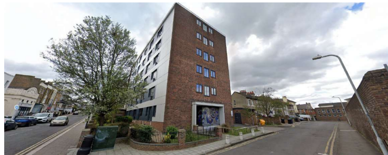
Zion Place Frontage
