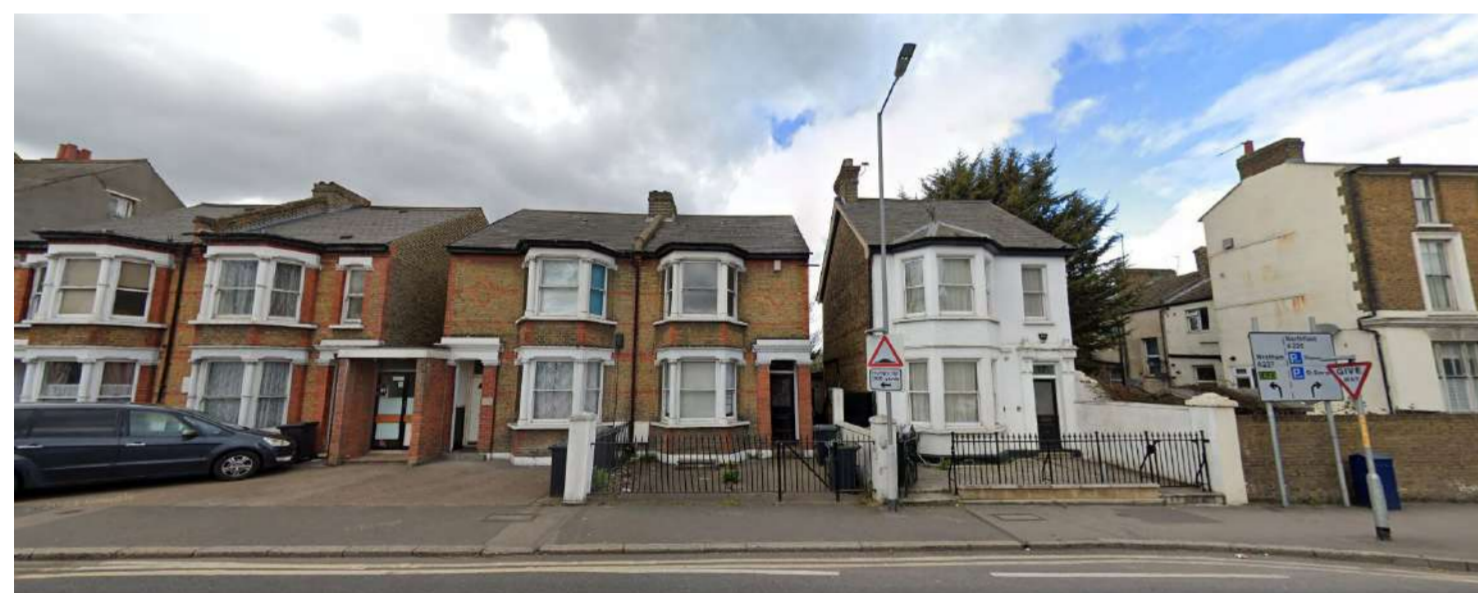
Wrotham Road Frontage
