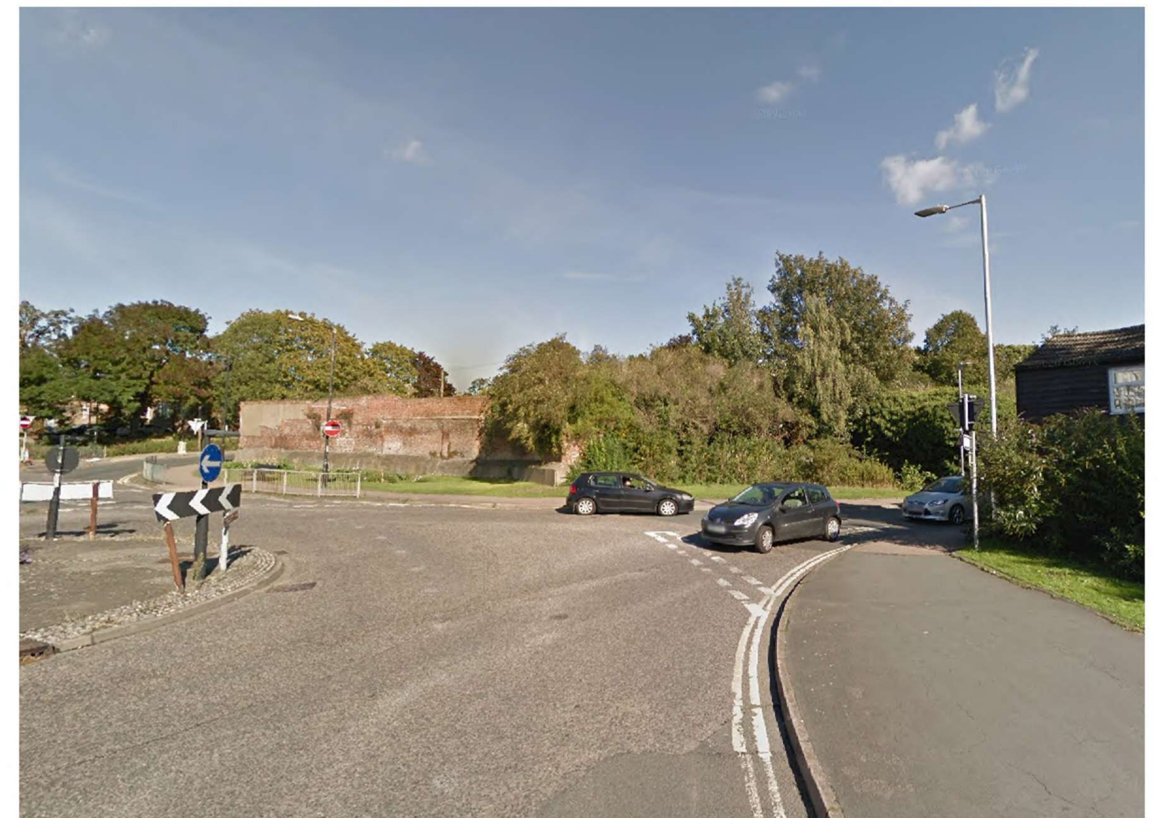
The existing application site enclosed on one side by an existing retaining wall
