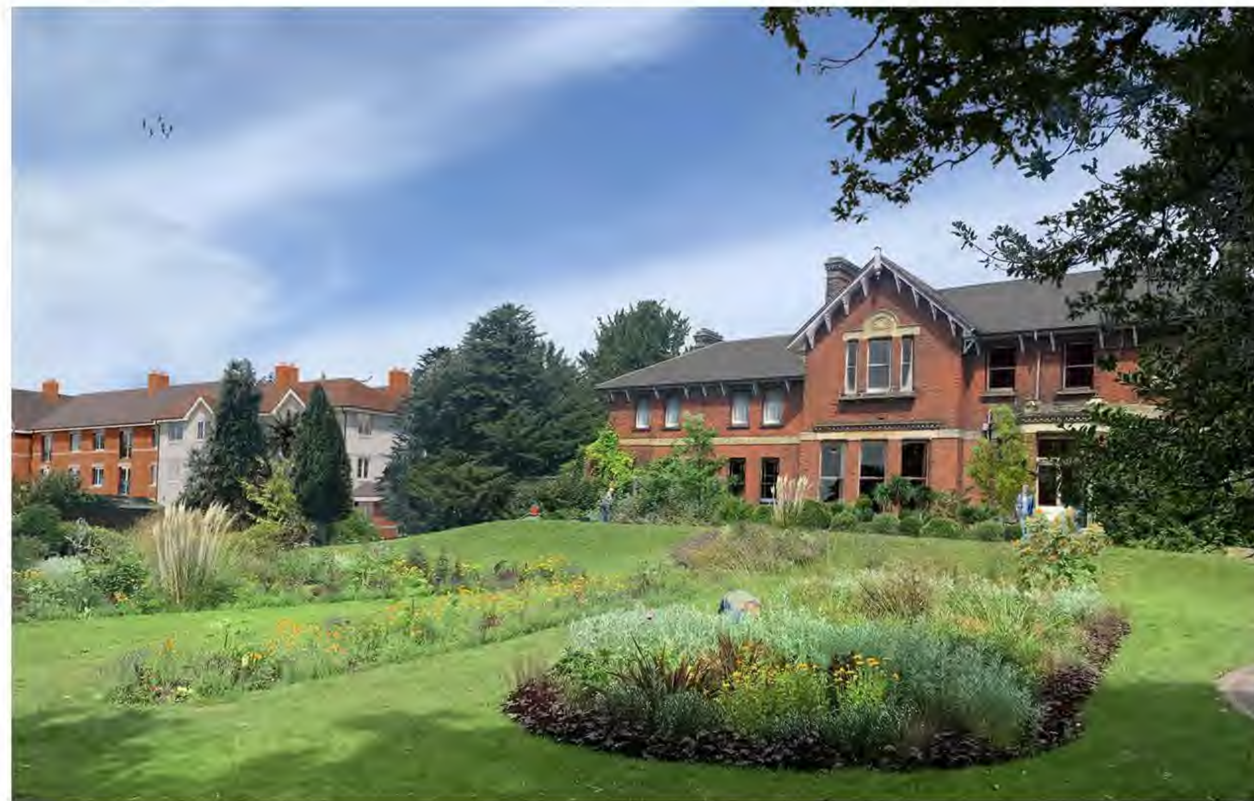
View of rear elevation from external garden amenity
